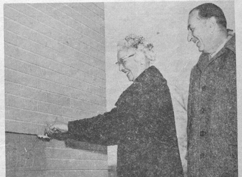
DR. MARION E. SHEA, Paterson State College president, and Dr. Kenneth B. White, dean of students, officiated at an informal cornerstone-laying ceremony on Friday, February 9. Two cornerstones were cemented — one in the new science-math-art classroom wing of Hunziker Hall, and the other in the new food service building. They are both dated 1960, the date of ground-breaking.
