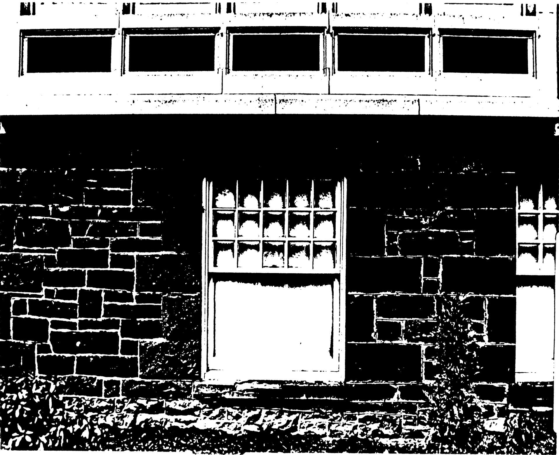
Illustration 12: Exterior Stonework Detail NPI photograph 1988
